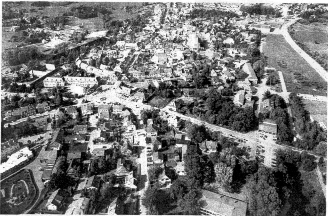
St. Vith Today: When compared with the pre-war photo, this recent aerial photo shows how large the rebuilt, "little city" has become. St. Josef's Klinik, successor to the Kloster, is in the left foreground with An den Linden traffic circle standing out beyond it. At the other end of town a commercial development has spread out over the open area through which the I&R came to temporary safety and reaches almost to the edge of what appears to be the draw which provided us with cover over to the lines of the 7th Armored Division.
