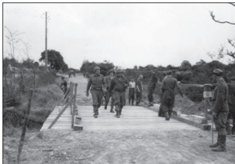
First patrol of infantrymen of the 106th Infantry Division (15th U. S. Army) crosses bridge built by Germans for passage of our troops at St. Nazaire, France, after surrender of the German garrison in the pocket of resistance. German bridge builders are at edge of bridge.
