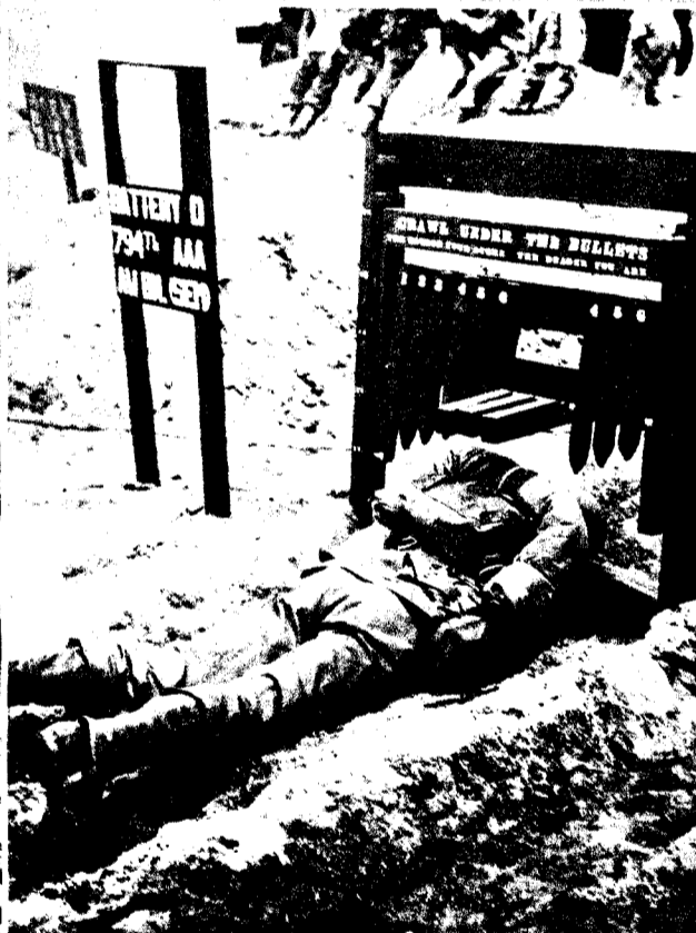
NO GUILLOTINE. It's an "infiltration trainer" at Camp Stewart, Ga., teaching soldiers to keep their heads down. If the crawler gets too high, the sticks touched register amount of exposure.
