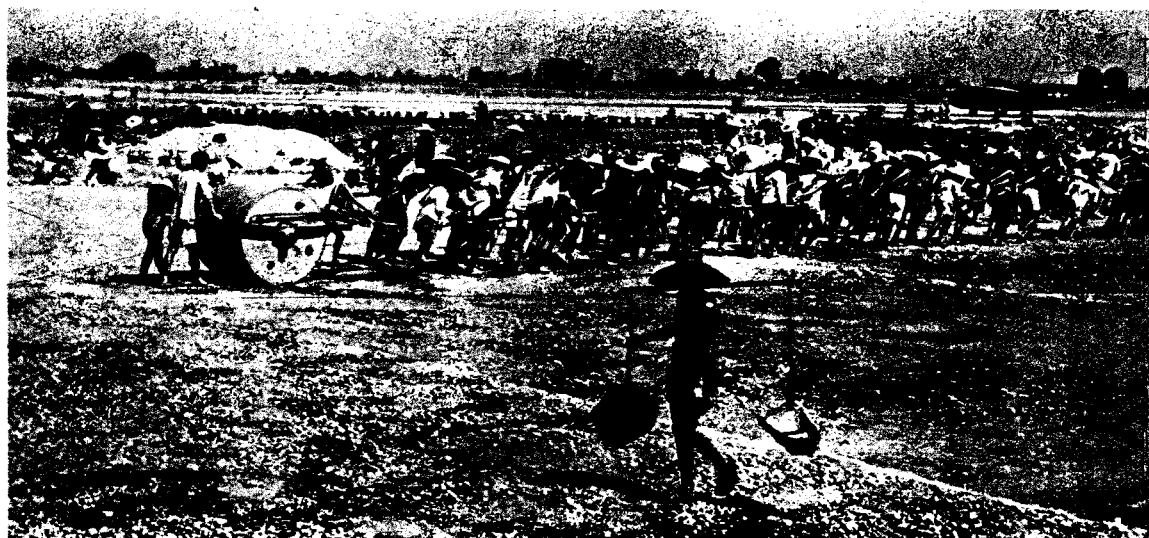
Thousands work to prepare the Superfort bases. Natives in construction crew tug on a mammoth 10-ton roller.
