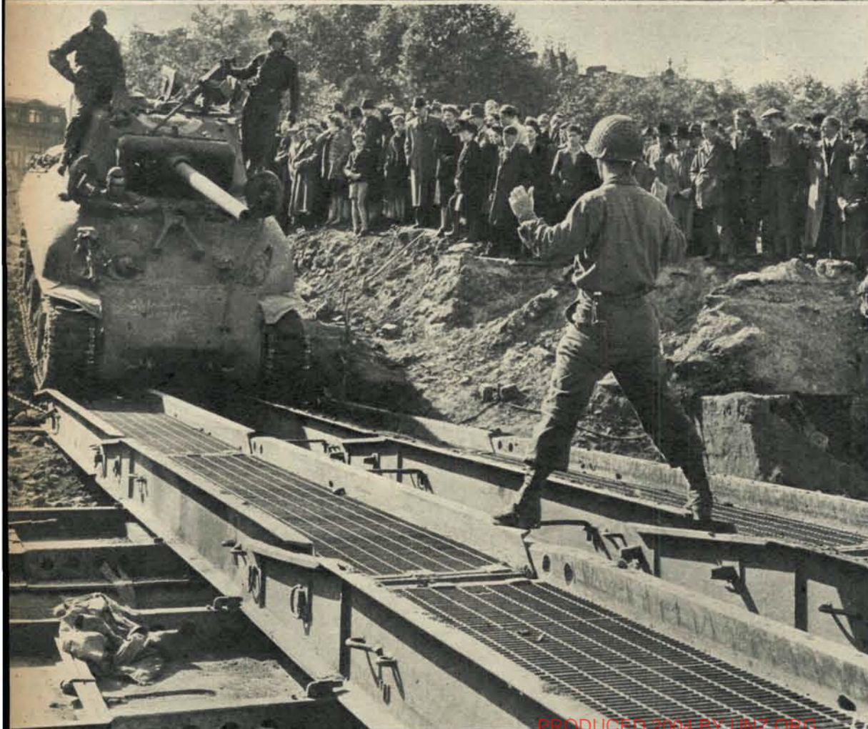
SHERMAN TANK ROLLS ONTO A PONTON BRIDGE BUILT BY AMERICAN ENGINEERS AT THE MEUSE NEAR LIEGE
