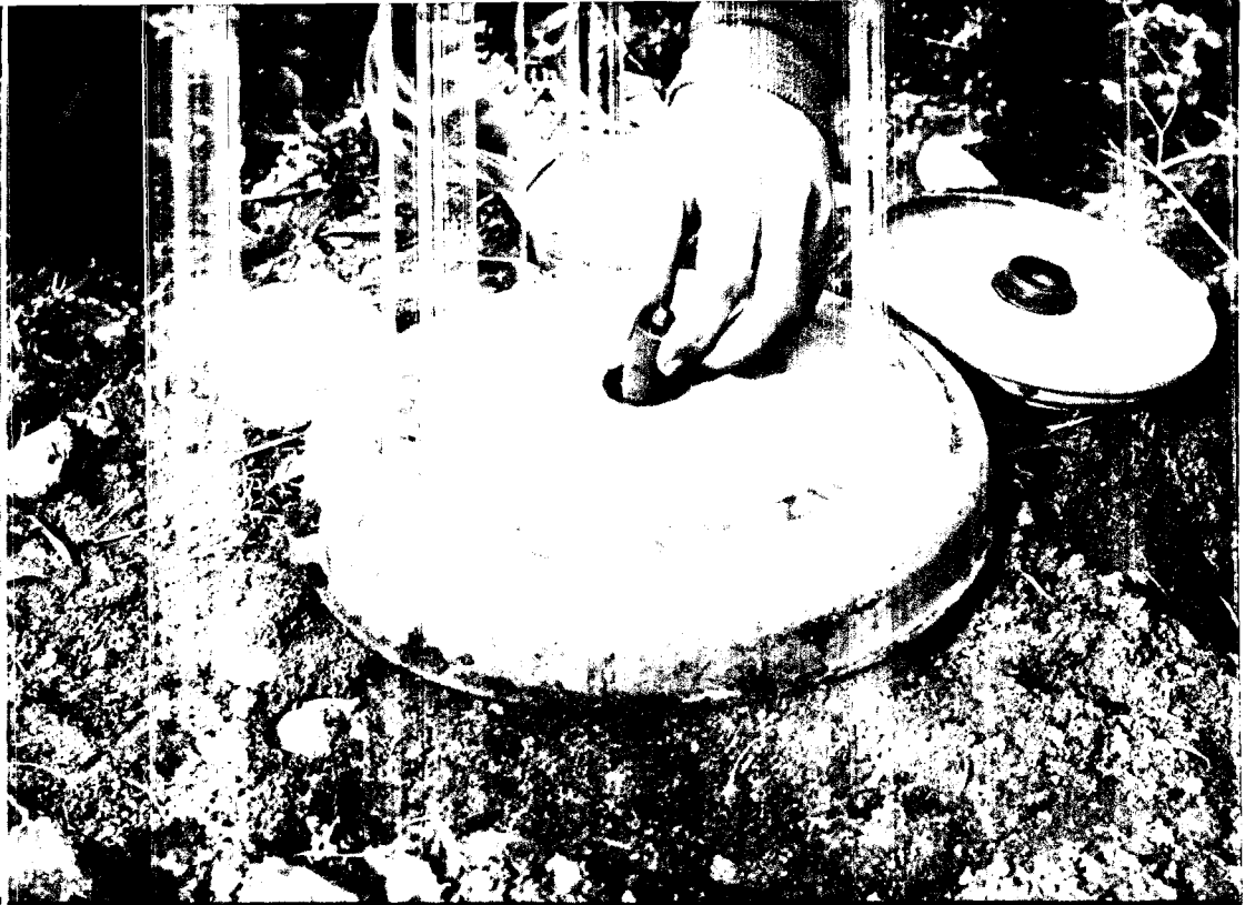
Soldier removes detonator from a Teller mine. The Teller mine is the most common type of German antivehicle and antipersonnel mine. They are often laid in open fields with narrow lanes, known only to the retreating Germans, leading a safe pathway through them for Nazi patrols.
