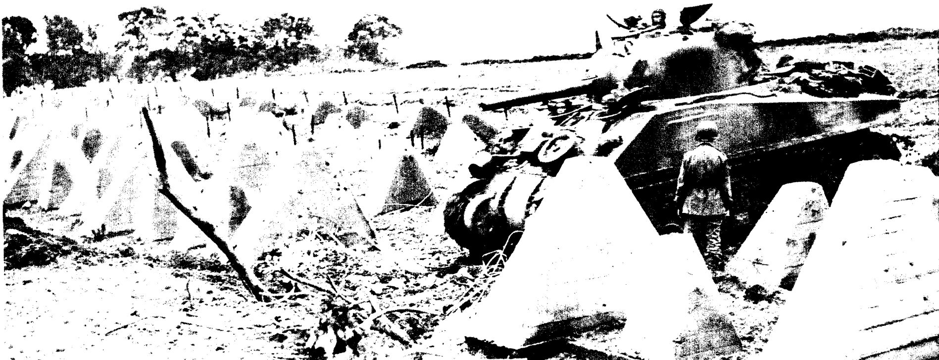
An M-4 Sherman tank moves through a belt of steel and concrete antitank obstacles in the Westwall. The path was created by engineers of a demolition squad.
