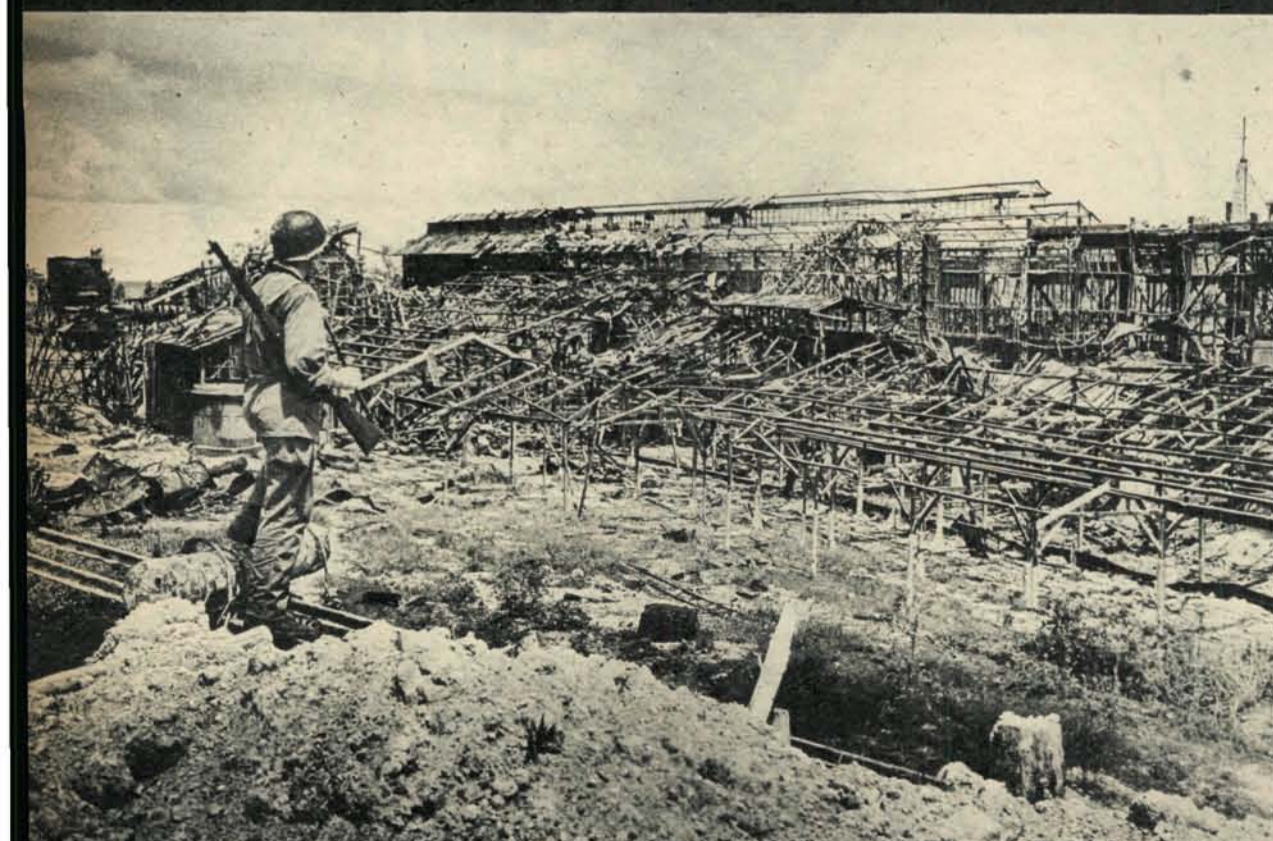
This is the way Jap phosphate plant on Angaur looked after the Navy and Army had finished with it.
